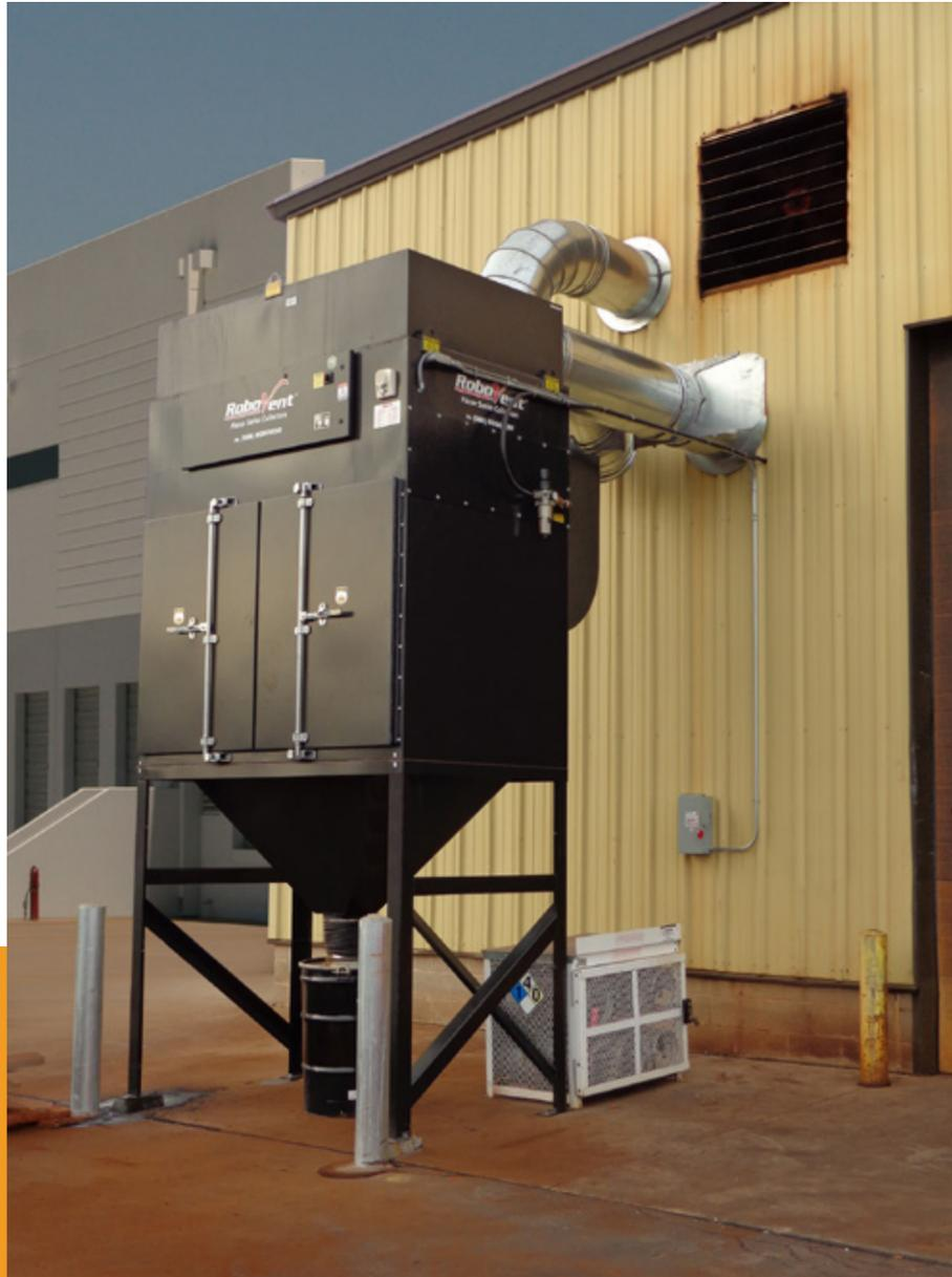
A high-powered, centralized dust collector can provide effective dust control for multiple laser cutting units.
